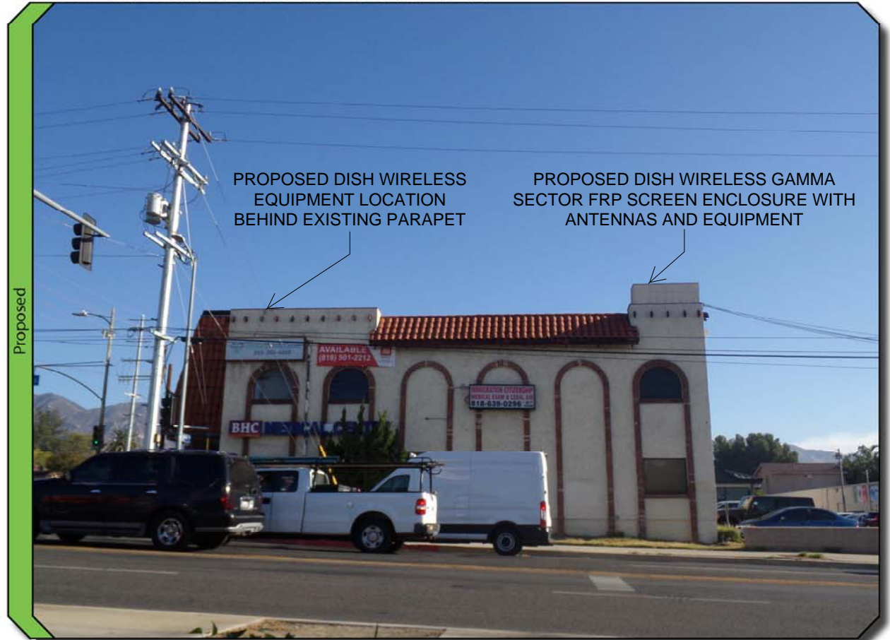
View 1 of 3: SOUTHWEST ELEVATION LOOKING NORTHEAST
