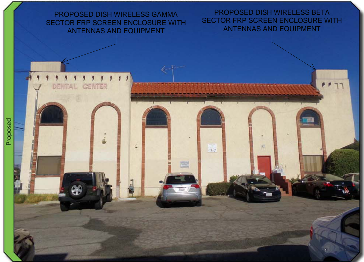
View 2 of 3: SOUTHEAST ELEVATION LOOKING NORTHWEST
